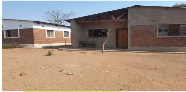
Two teachers houses constructed by the community.
